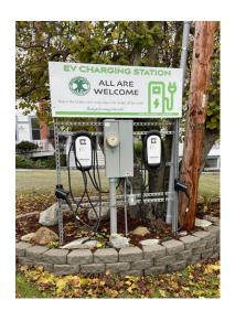
\*\* This is the configuration of the EV charging station at First Presbyterian Church, Port Townsend, WA. Pole/pedestal outside in the parking lot. These chargers are manufactured by ClipperCreek (HCS-60 EV Charger 48A With SAE J1772 Connector). The cost for this installation was under \$4,000. [Note ClipperCreek and Enphase are now the same company]. The electricity cost for this configuration in Fairfax County would be about \$0.45/hr., the same as providing an electrical outlet (option 1).
