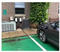
\*\*This is the configuration of the EV charging station at Peace Church in Fairfax City. These chargers were installed in 2019 and cost about \$730 each. Built for extreme weather conditions and high-traffic use with a 5-year limited warranty. Wall mounted. The manufacturer is Enphase and the model is HCS-40 EV (32 A, 7.7 kW, hardwired). The location of the charger is discoverable on Plug Share. Unique to this installation is that the chargers draw power from the church solar roof panels.
