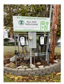
\*\* This is the configuration of the EV charging station at First Presbyterian Church, Port Townsend, WA. Pole/pedestal outside in the parking lot. These chargers are manufactured by ClipperCreek (HCS-60 EV Charger 48A With SAE J1772 Connector). The cost for this installation was under \$4,000. [Note ClipperCreek and Enphase are now the same company]. The electricity cost for this configuration in Fairfax County would be about \$0.45/hr., the same as providing an electrical outlet (option 1).
